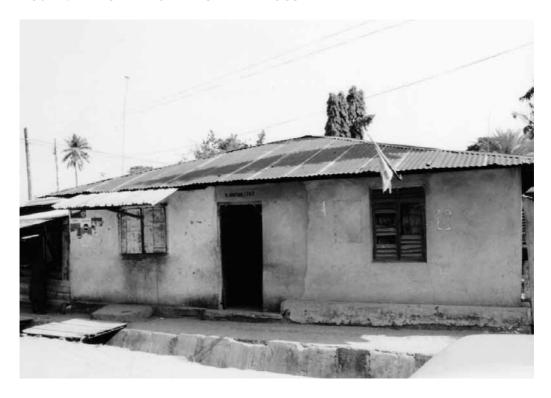
The modern Swahili type in Dar es Salaam is usually built with a proper foundation made of concrete or other durable material such as stone, its walls are made of sand cement blocks and the roofing cover is iron sheets. In the recent years, roofing tiles have also become a common roofing material.
