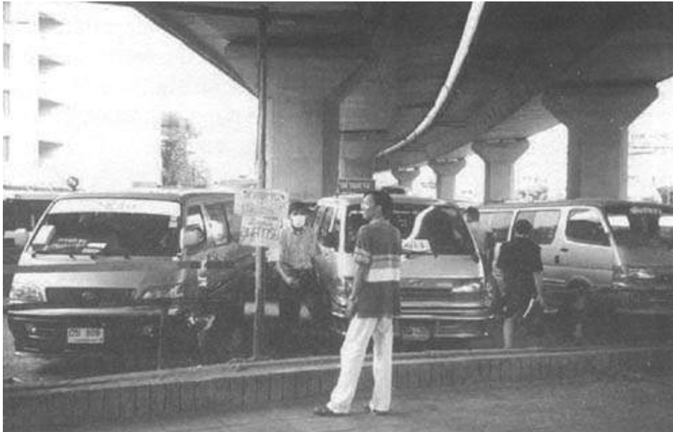
Photo 4.3. Vans Queue Under Freeway Right of Way Near Victory Monument
