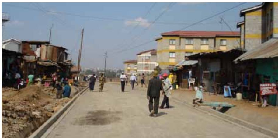
FIGURE 3.1: New 12m road Kibera - labour based construction
