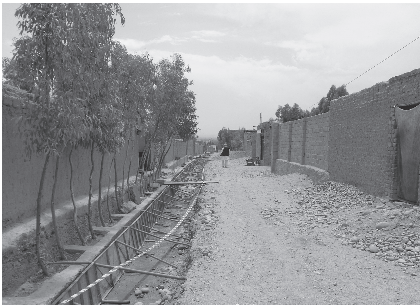
Picture 30: Drainage infrastructure under construction, Qasamabad Damankalil
