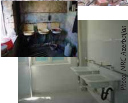
Bathrooms before and after upgrade
