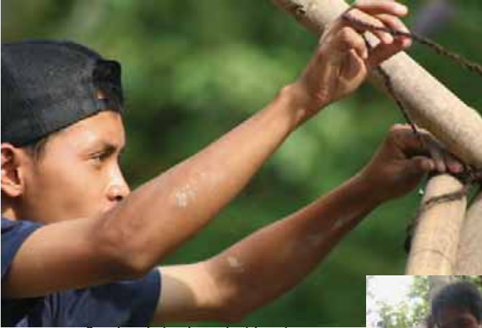
Bamboo being bound with string
