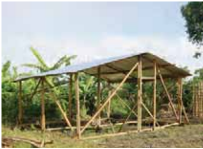
Structural skeleton of a house, showing cross-bracing
