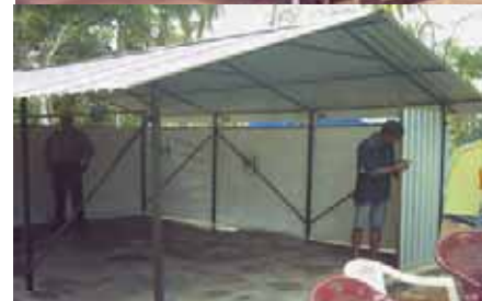
The construction of the shelters was not a difficult process.
