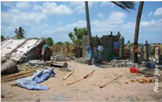
Core shelter under construction
