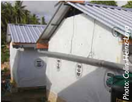
Shelters built with tanks for rainwater harvesting
