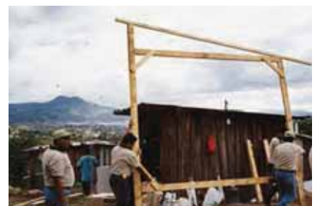
Shelter assembly using prefabricated walls
