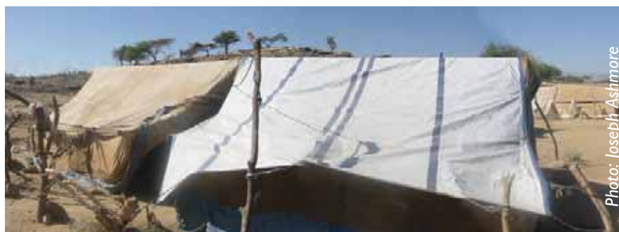
A fly sheet separated from an inner tent and covered with plastic is used to form an extension. Sticks were used to raise the sides to increase the internal volume.
