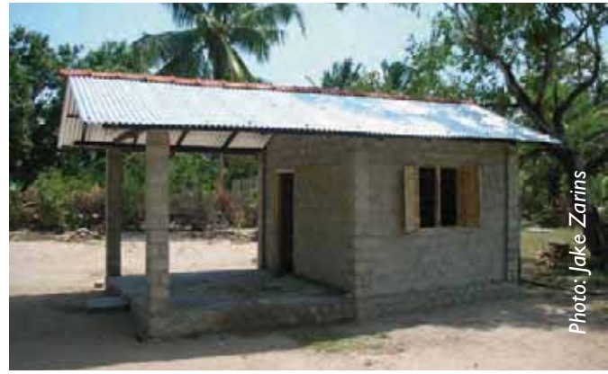
Completed core shelter
