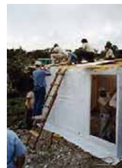
Covering the roof with corrugated iron
