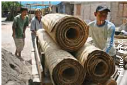
Transporting bamboo mats to a construction site
