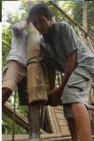
Connecting a vertical post to the foundation
