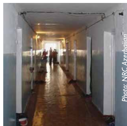
Corridors before and after upgrade
