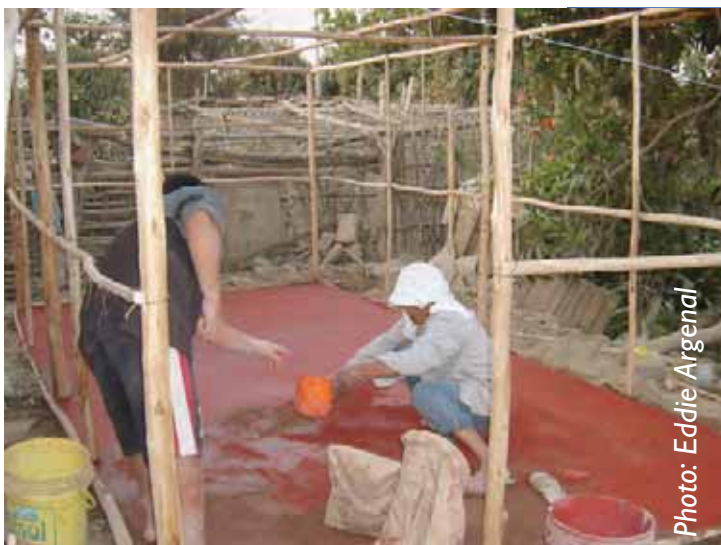
Making the concrete floor slab
