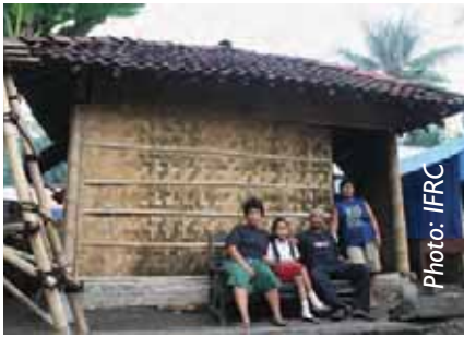
A completed transitional shelter built through cash grants
