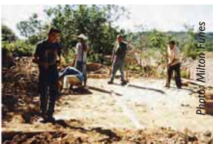
Marking out the site for a shelter
