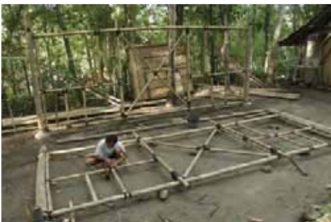
Prefabrication of a wall panel
