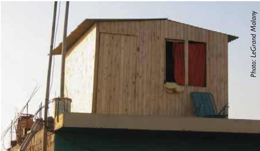
Completed shelter built on the roof of a damaged house
