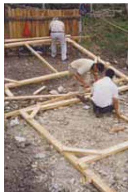
Prefabricating walls
