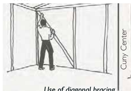
Use of diagonal bracing
