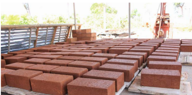
CSEB production at the MN/ Ikra Government Muslim Mixed School construction site.
