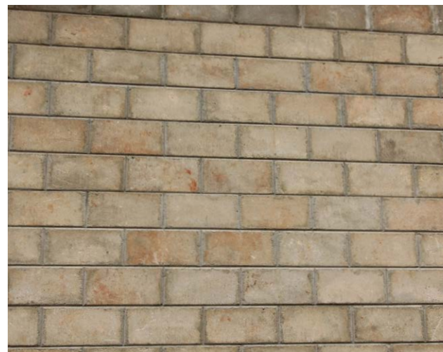
Wall constructed using fair-faced masonry.
