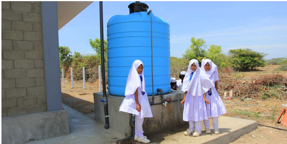
WASH facilities for girls at Periyapandivirichchan Primary School and RWH system and water tank at Koolankulam Government Muslim Mixed School.
