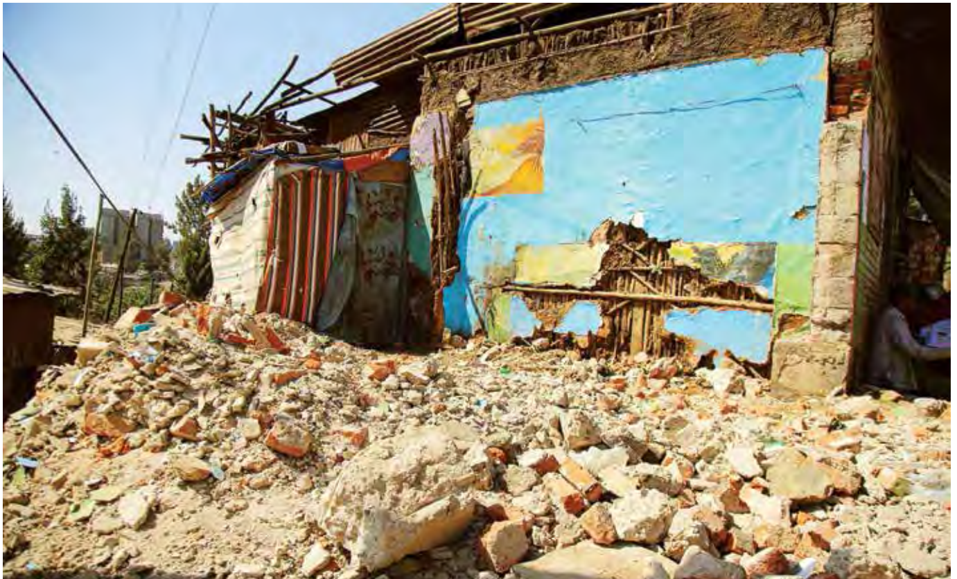
▲ Half demolished Kebele house. © Geo Kalev.
