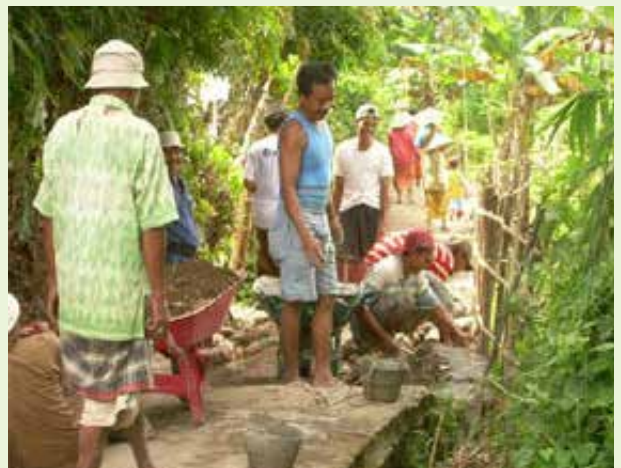
Street construction by residents. Photo: Asian Development Bank
