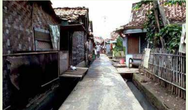
Street after upgrading. Photo: Marc Jansen
