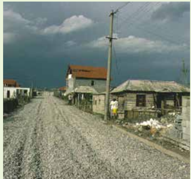
Defining the public space allocated to streets in Bathore informal settlement through gravel pavement, Tirana, Albania. © Coplan.
