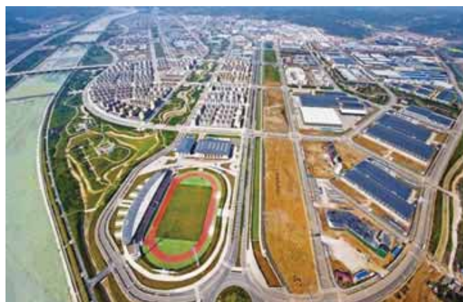
Aerial photo of new Beichuang City
