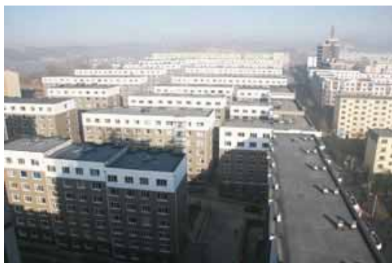
Jiumalu Road, Xiangyang District after energy conservation upgrading
