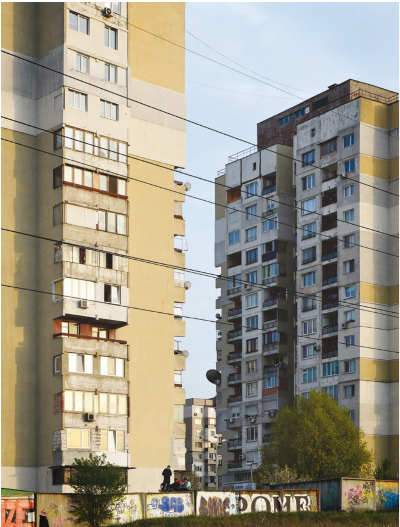
Refurbishments funded by the European Regional Development Fund are being carried out for buildings in Sofia with the lowest energy efficiency
