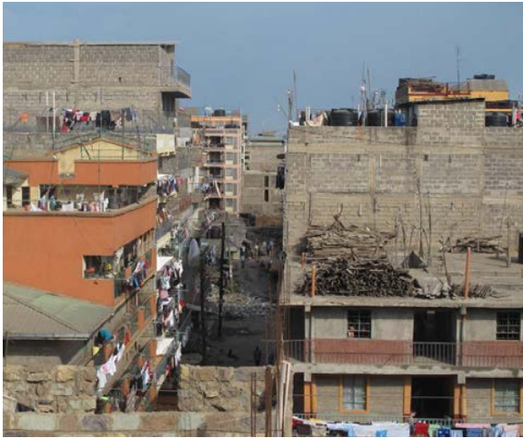
Incremental Tenement Construction in Embakasi, Nairobi © Baraka Mwau
