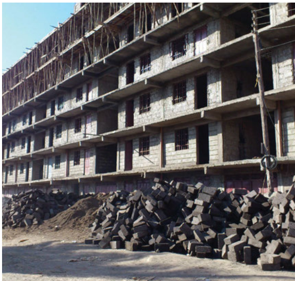
Building construction in Embakasi, Nairobi © Baraka Mwu
