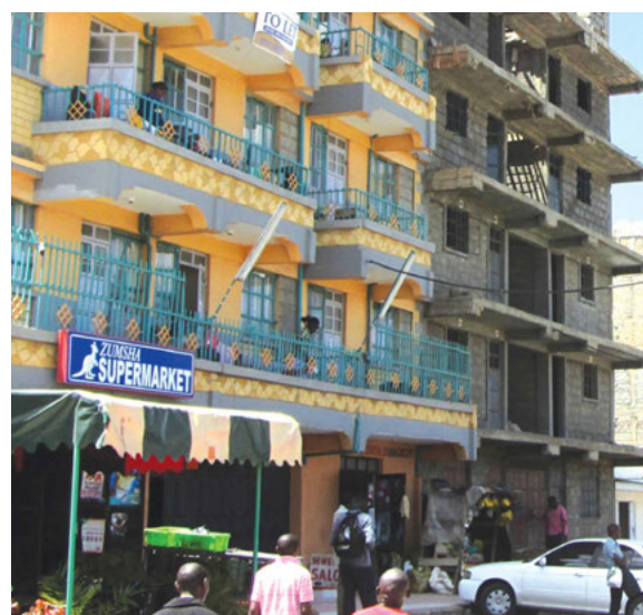
Mixed-use developments, Embakasi, Nairobi © Baraka Mwau
