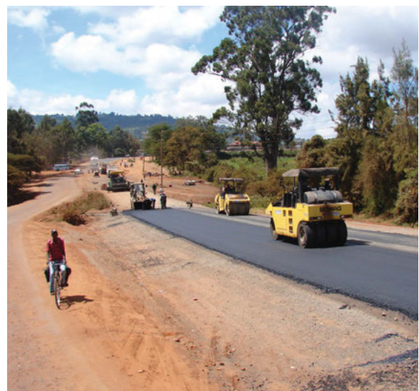
Road construction in Kenya © Flickr/computerwhiz417
