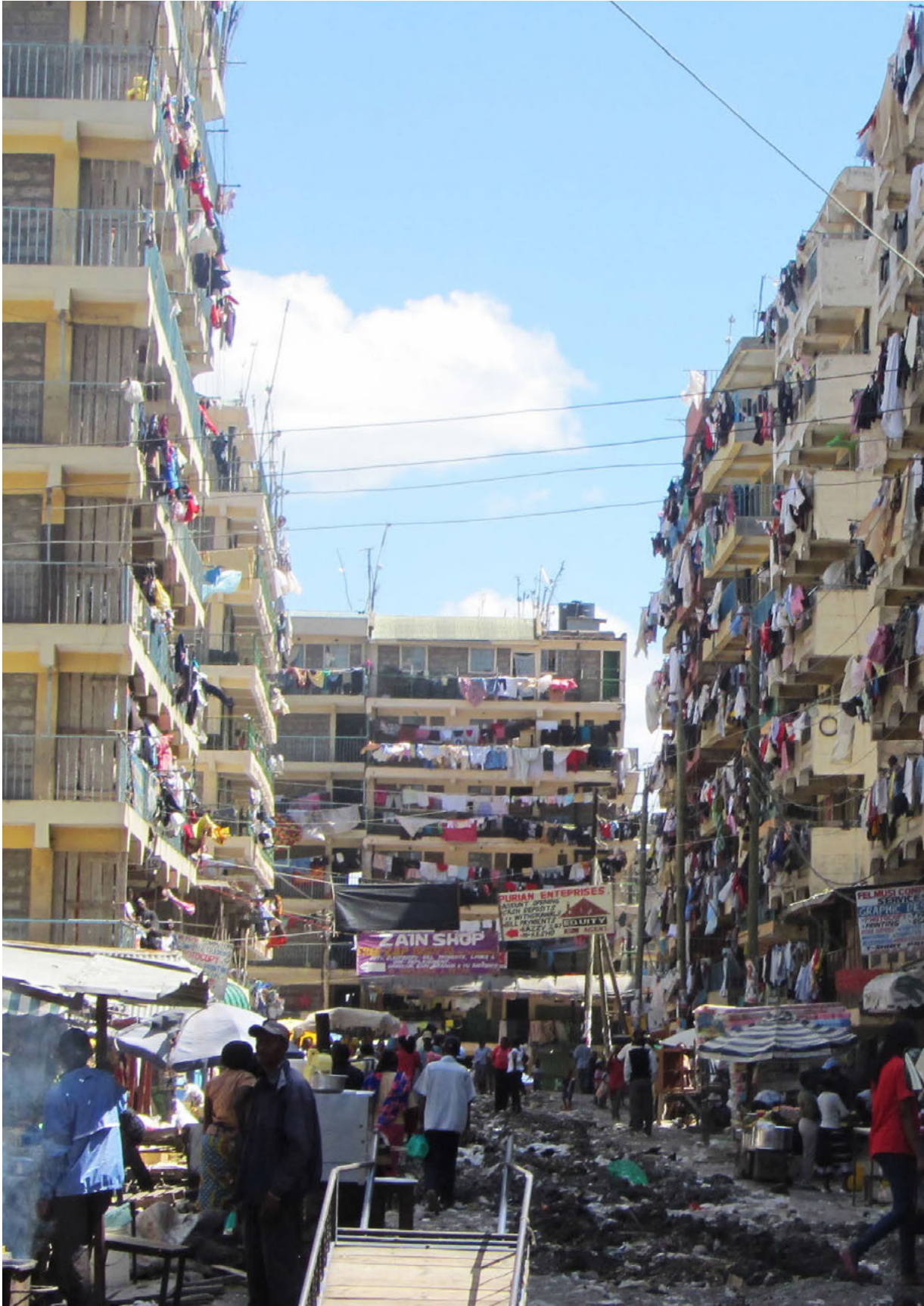
Tenement Housing in Embakasi, Nairobi © Baraka Mwau
