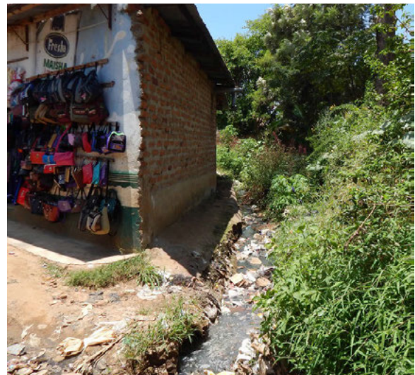
Drainage challenges in Kitui © Baraka Mwau
