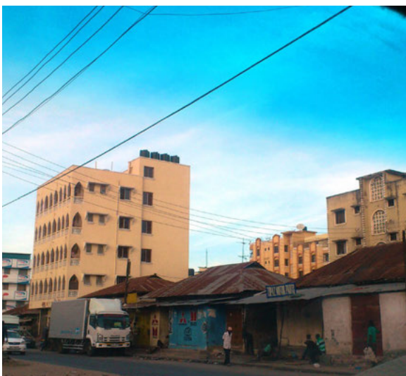
Housing redevelopment in Mombasa © Baraka Mwau
