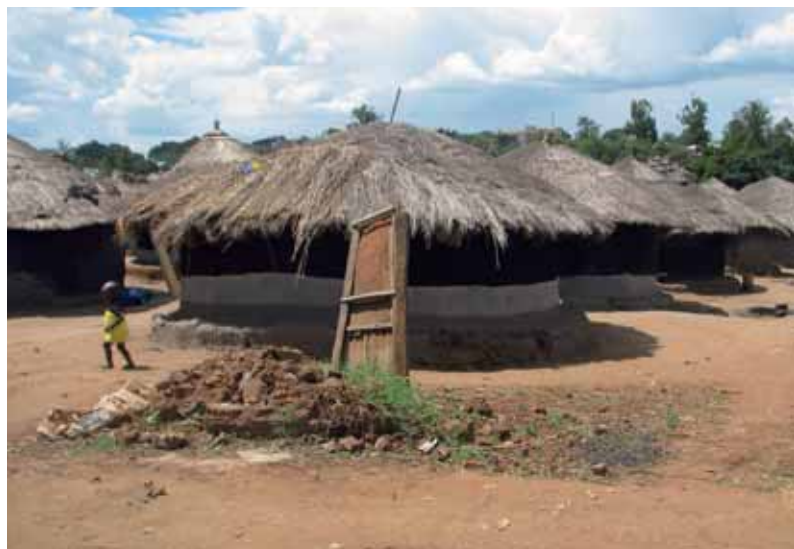
Figure 3. IDP Housing in Gulu. © Vincent Ahimbisibwe
