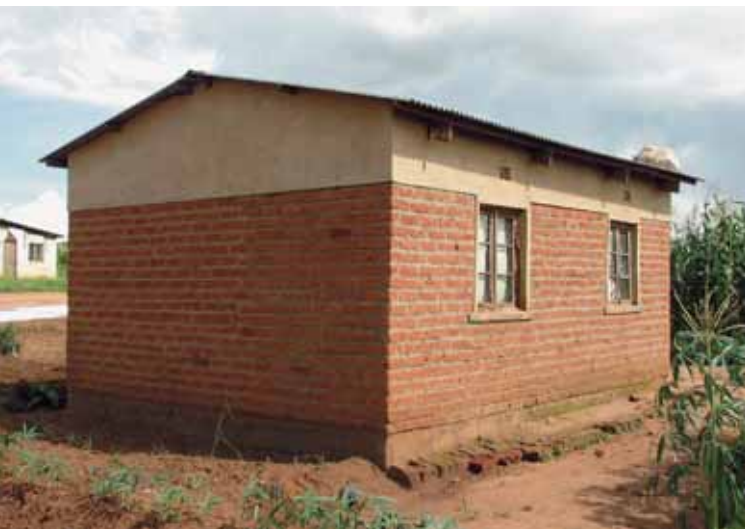
Figure 27. A house constructed with burnt bricks. Photo © Martin Kaggwa
