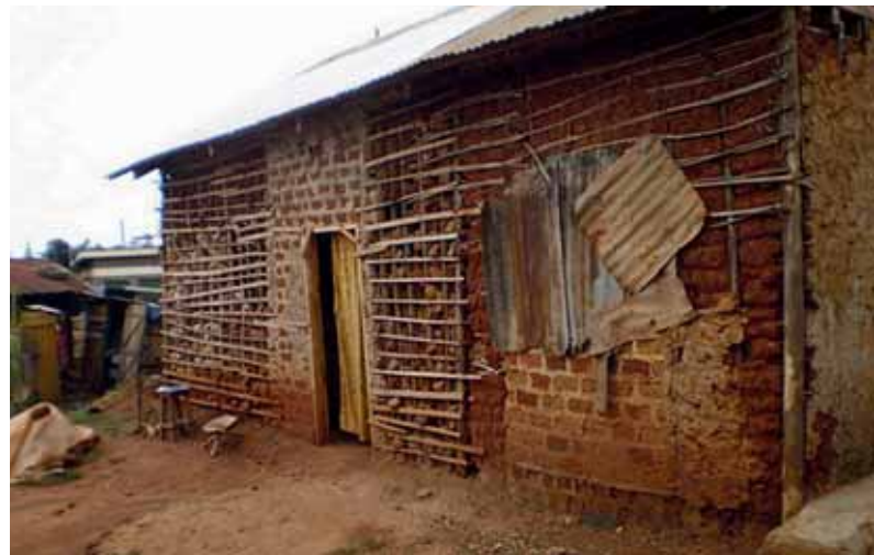
Figure 11. Incremental building with mixed materials and limited fixed infrastructure in Kampala's informal areas.
