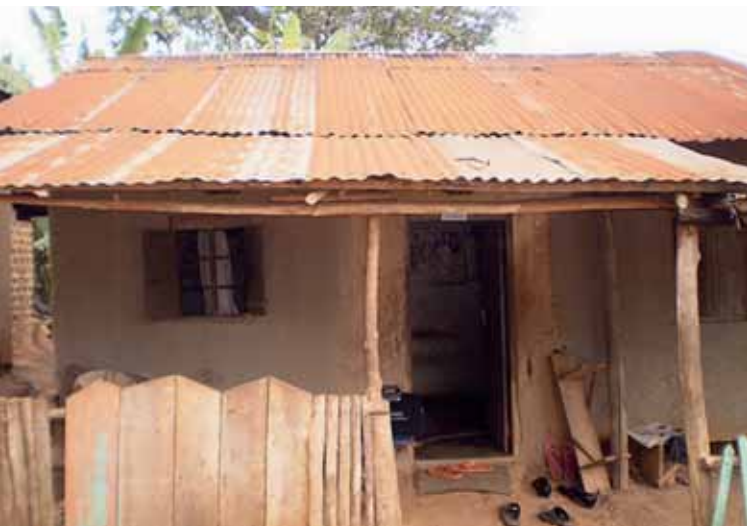
Figure 13. Tin-roofed home on formally registered plot in Kampala. © Martin Kagawa
