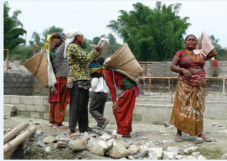
Women constructing their new homes, Lumanti, Nepal. © Lumanti
